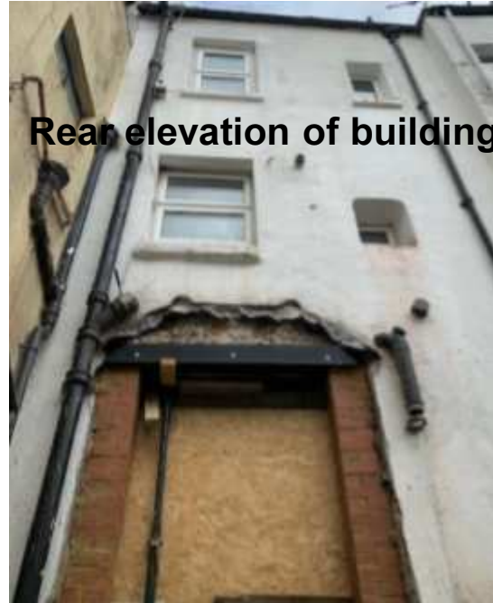
View north east from rear patio towards rear of 22 Trafalgar Street
